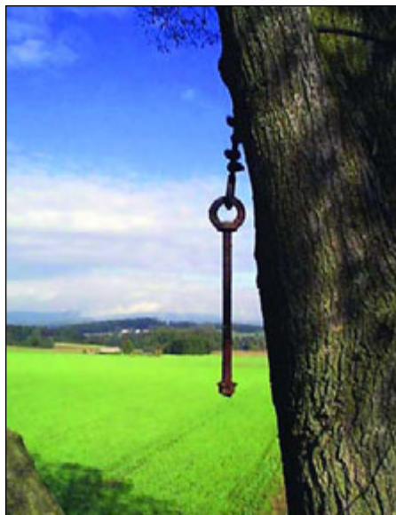
Pull-out failure of a through-bolt.
